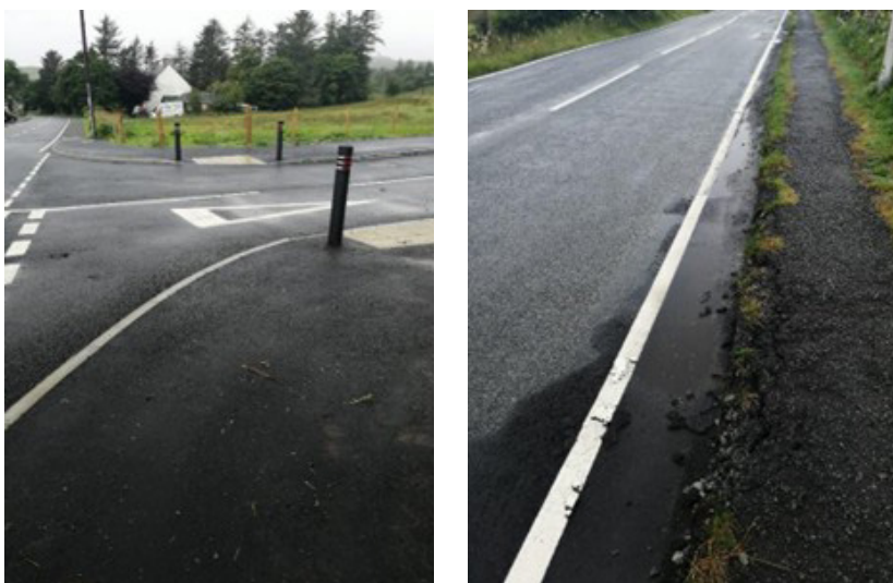
Dunvegan pavement contrast: Modern pavement at Dunvegan Primary School vs pavement from Lonmore-Dunvegan with wooden curb.
